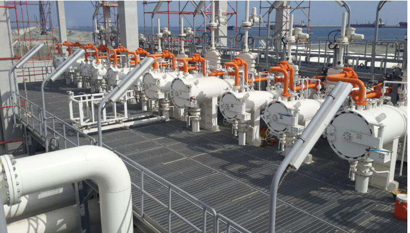
VKVC Launcher with Mobile Pig Handling System suitable for various size Pipelines
